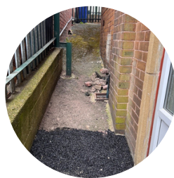
After the leak was fixed
